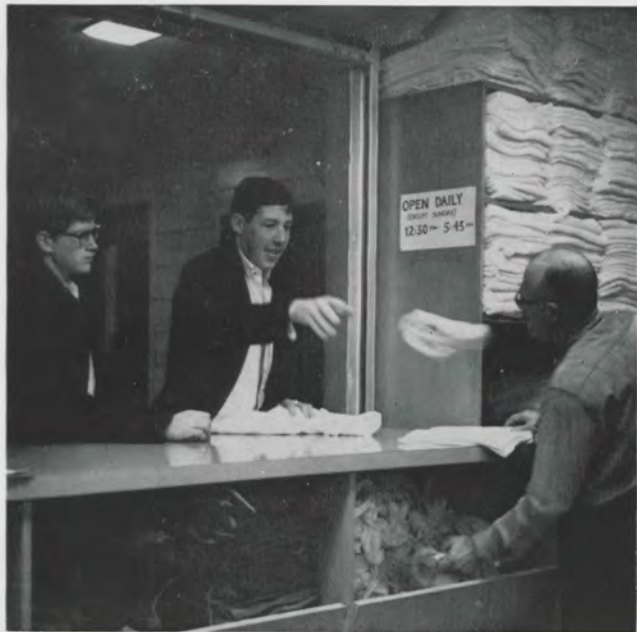
The new facilities are complete: a stock-room . . . .
